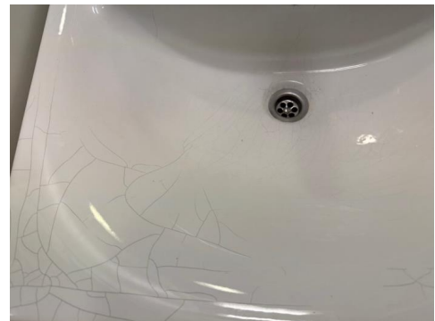
Riss/krakelering i servant.
